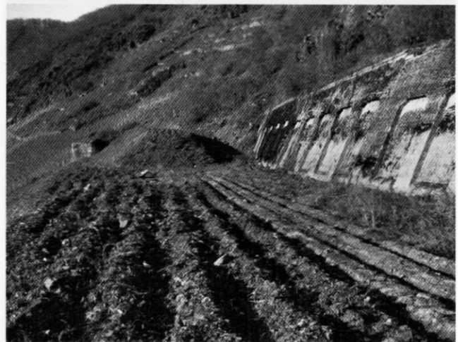
Simulated view of the Bruttig (south) portal in March 2011. Photo by Peter Jigins
